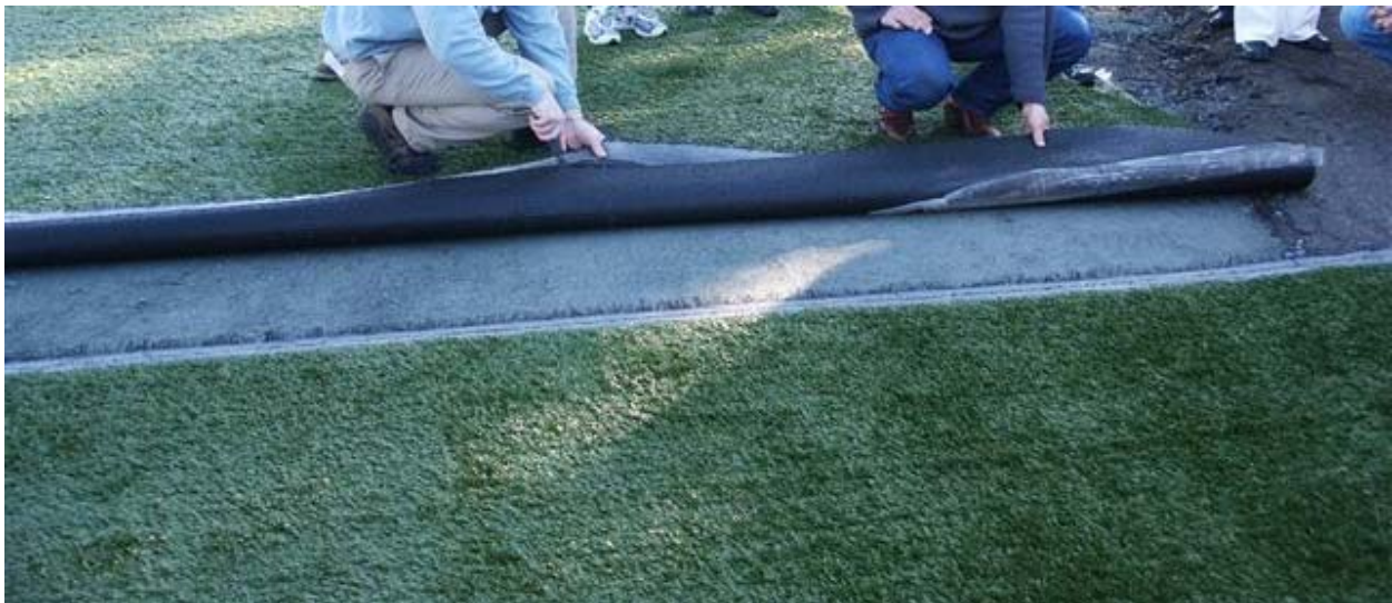
Turf is laid down over the aggregate and weed barrier and glued at the seams before securing to the ground. Photo from Soquel Creek Water District
